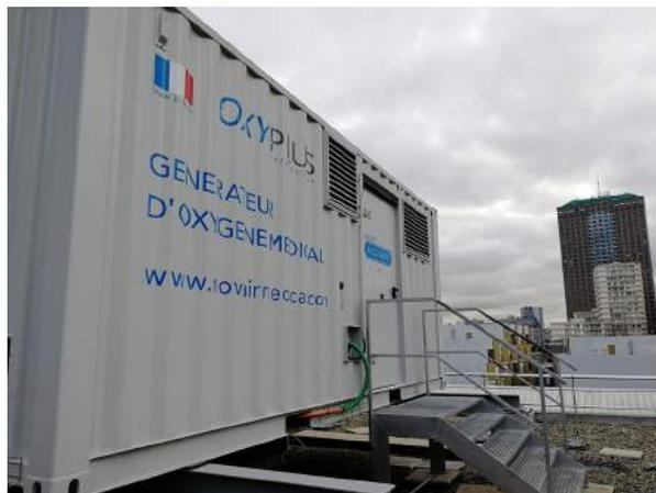
Caption : Containerized PSA oxygen plant installed on the roof of La Roseraie Hospital near Paris, France
