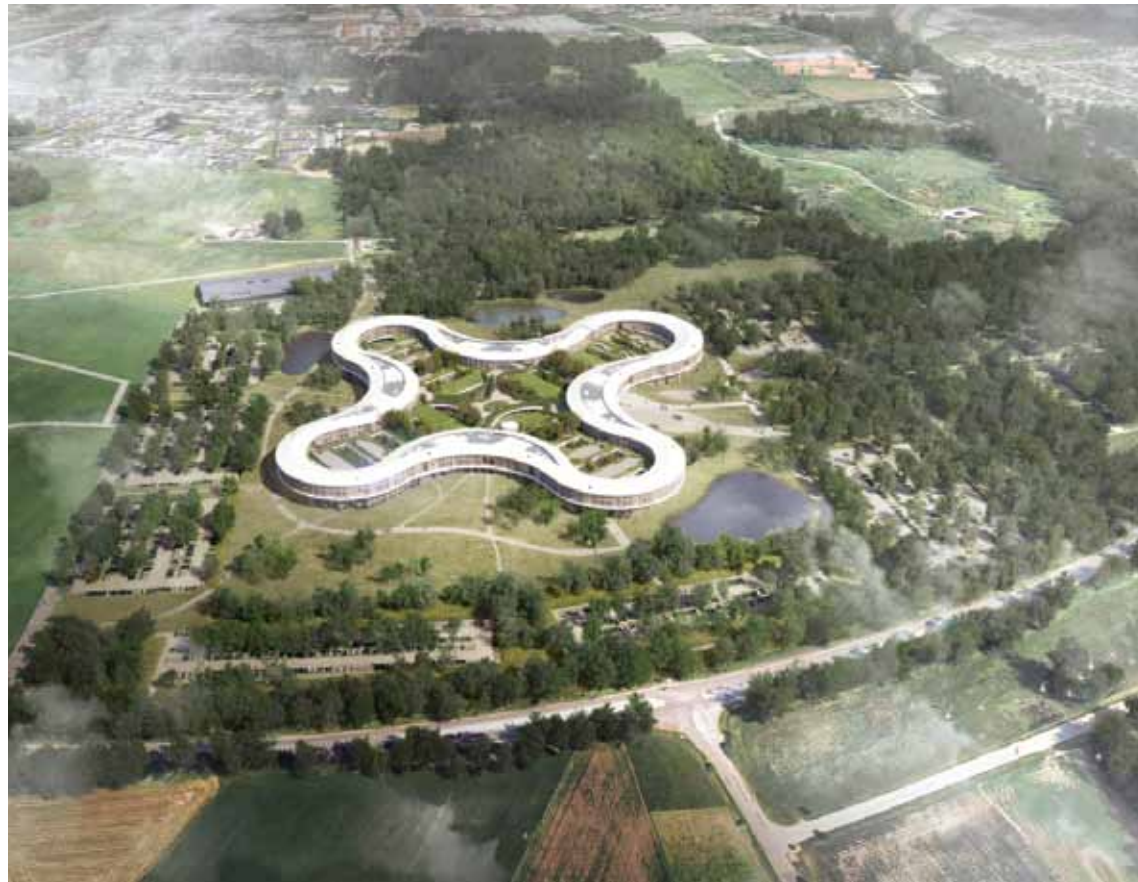
Figure 3. Nyt Hospital Nordsjælland by VLA with Herzog & De Meuron Architects – Aerial.
